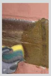
After that, fill the defect and remove excessive material with a sponge. A dry brush is well suited to clear the wood structure.
