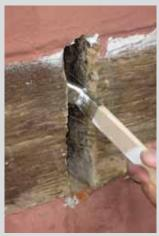
The defects are primed with the liquid component 24 hours before refilling. Then the cut fitting piece or wedge is fit centrically into the void with the wood filler KEIM Lignosil-HRP.
