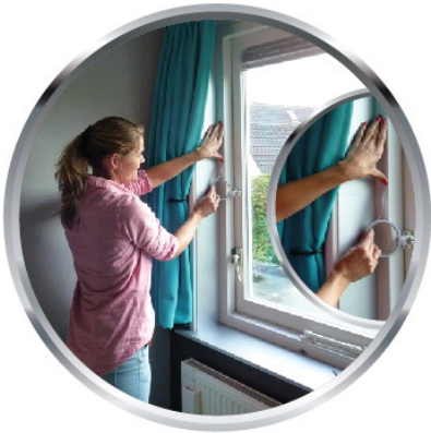
1. Place the adhesive tape around the window frame
