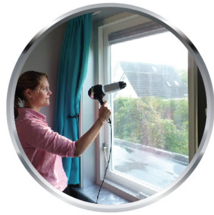
3. Shrink the film by hot air using a hairdryer
