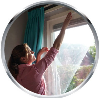
2. Attach the film to the adhesive tape
