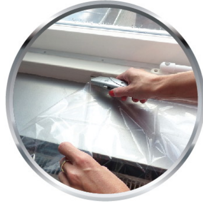
4. Cut off the remaining parts of the film
